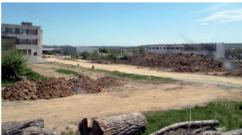
Fig.6.: Planá – airport complex. Position of construction of the road and laying of the water supply, (Photo by T. Pancíř). Overburden as part of landscaping, related to the construction of the hall – a building in the distance
