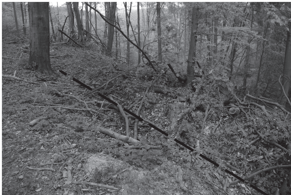
Fig. 1 Photographs of the current state of the Russian trench at elevation 500. The dashed line marks the bottom of the trench (by J. Zubalík).
