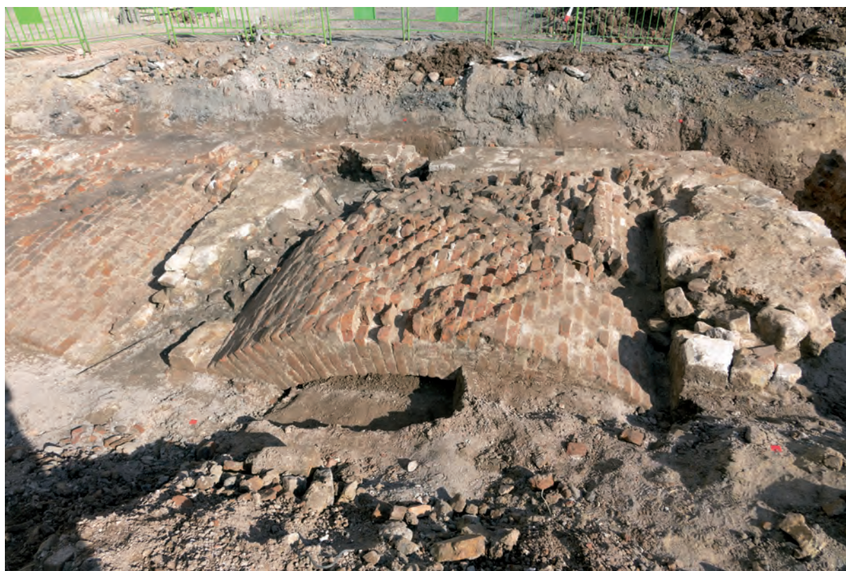
Fig. 19. Gayer's Barracks, extension of the building of the Museum of East Bohemia, a view from the west on the front wall of the rampart reinforced with pillars connected by vault arches, 2019 (Archive of the Museum of East Bohemia in Hradec Králové).
