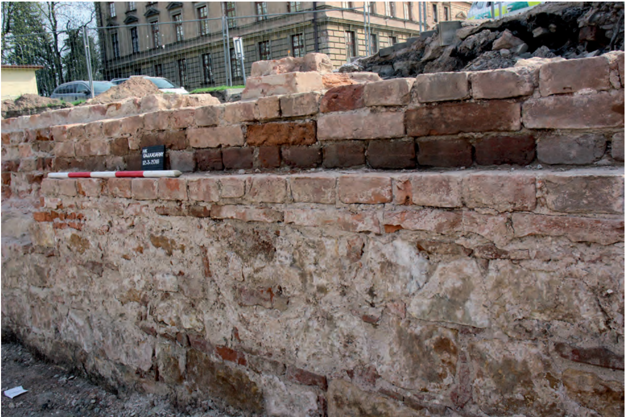
Fig. 13. Gayer's Barracks, uncovered relics of cavalier XXXIII, detail of one of the foundation walls with preserved rows of the original aboveground masonry, 2018 (Archive of the Museum of East Bohemia in Hradec Králové).
