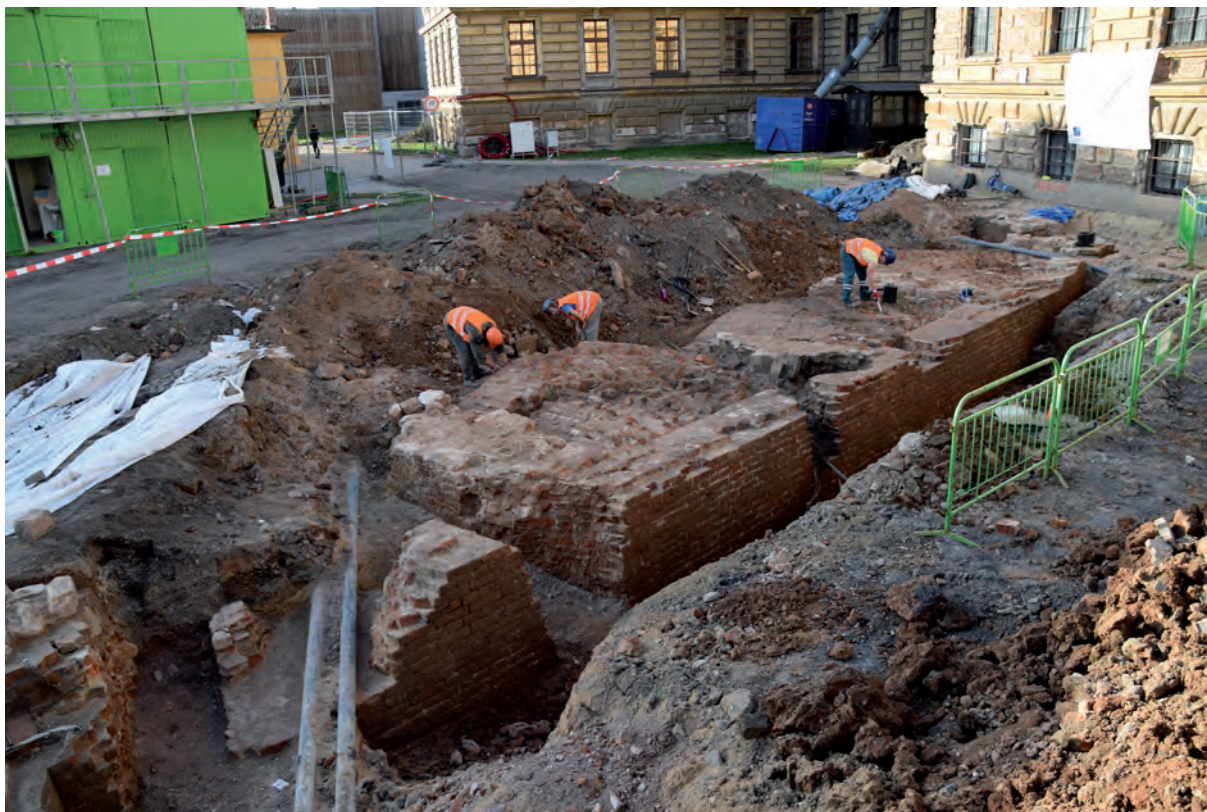
Fig. 17. Gayer's Barracks, extension of the building of the Museum of East Bohemia, a view from the southeast on the brick face of the front part of the rampart with visible interchanging of rows of stretchers and headers, 2019 (Archive of the Museum of East Bohemia in Hradec Králové).
