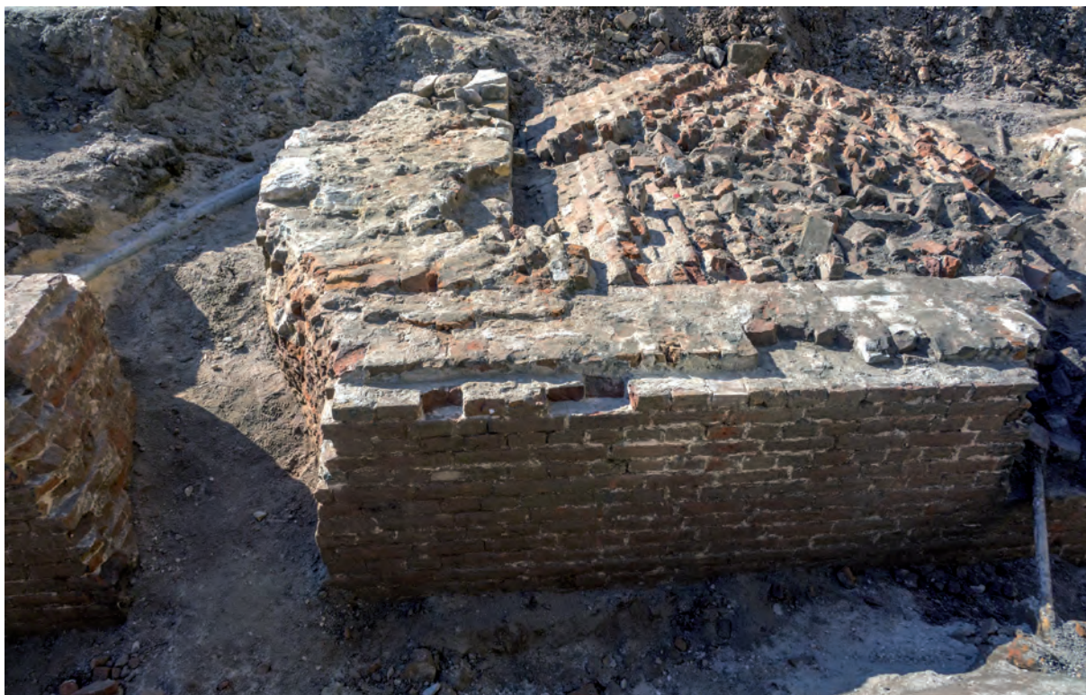
Fig. 18. Gayer's Barracks, extension of the building of the Museum of East Bohemia, a view from the southeast on the brick face of the front part of the rampart with visible interchanging of rows of stretchers and headers, detail, 2019 (Archive of the Museum of East Bohemia in Hradec Králové).
