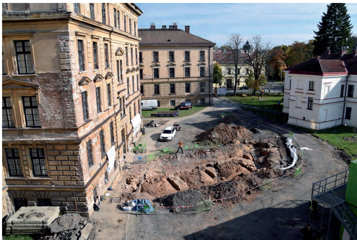
Fig. 15. Gayer's Barracks, extension of the building of the Museum of East Bohemia, excavation of foundations of the eastern part of bastion VIII, a view from the west, 2019 (Archive of the Museum of East Bohemia in Hradec Králové).
