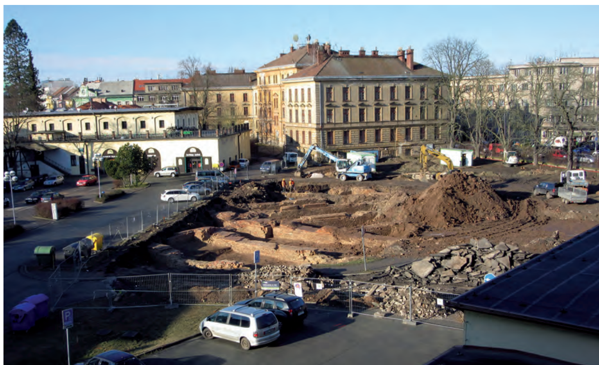
Fig. 10. A view from a window of the building of the Museum of East Bohemia (house No. 334) on the uncovered foundations of one part of cavalier XXXIII, 2018 (Archive of the Museum of East Bohemia in Hradec Králové).
