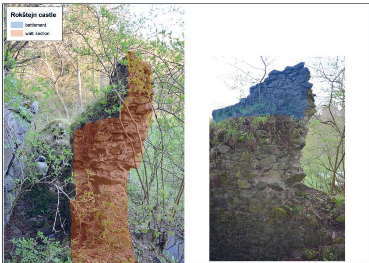
Fig. 10: Rokštejn, western Zwinger, Zwinger wall (part 2b on Fig 9) with a wall walk and battlement, see the narrow space between the rock and the wall, and relatively low height above modern terrain of 2,5 m.
