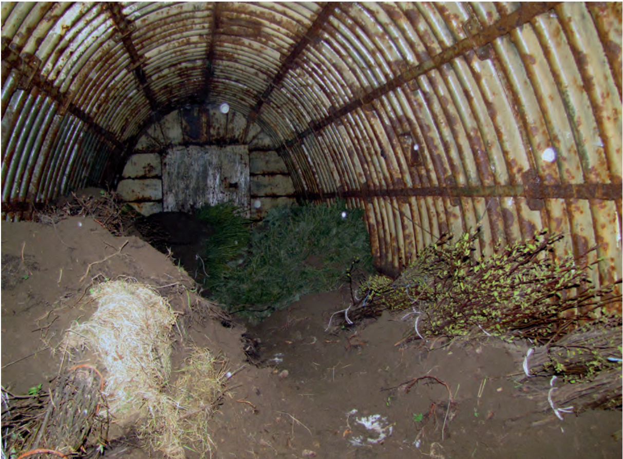
Fig. 28 – Hluboká u Trhové Kamenice (Chrudim District), emplacement for a battery of mobile rocket forces with shelter, 1970s–1980s. A view into the shelter interior. Situation as in 2014. Photo J. Musil.
