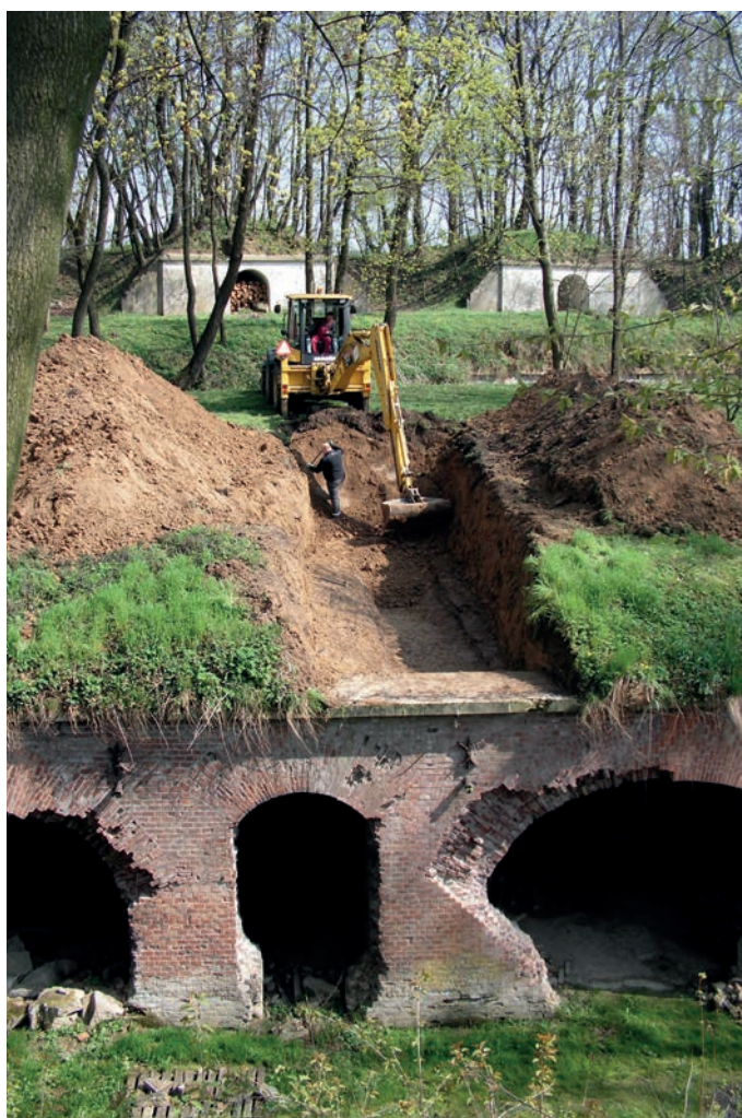
Fig. 20 Dumping of secondary layers over the western shoulder of the central casemate block.
