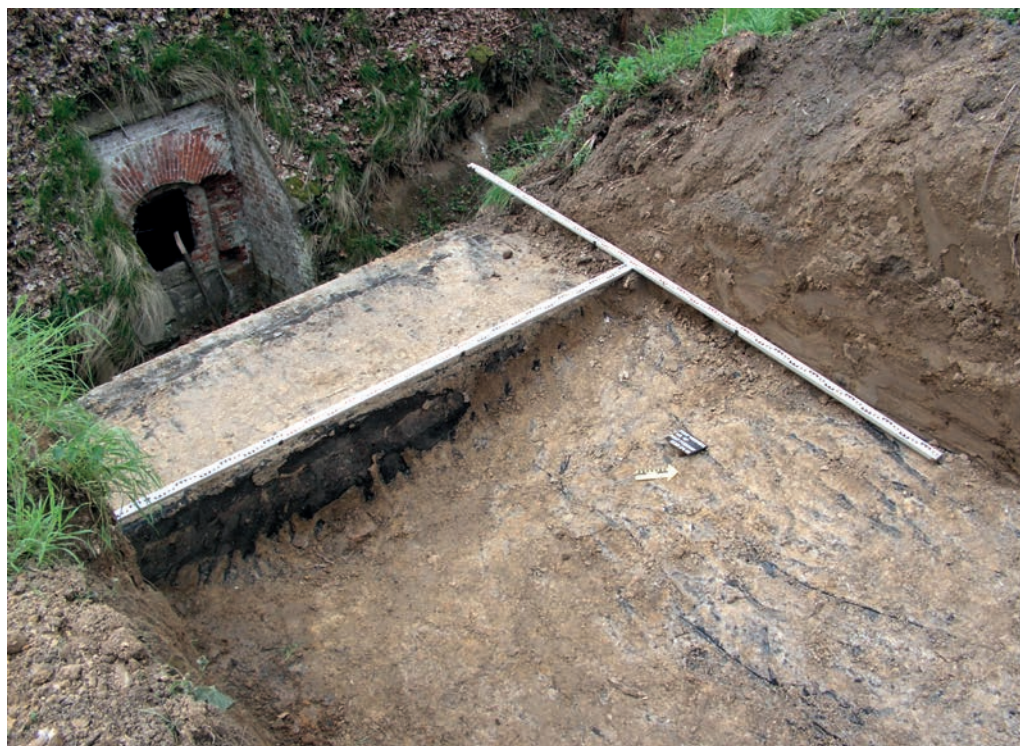
Fig. 22 View of the cornice.
