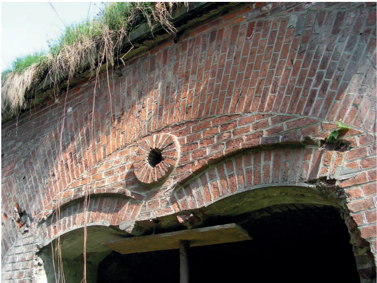
Fig. 16 Elevation bricks above the entrance to the central casemate block – detail.
