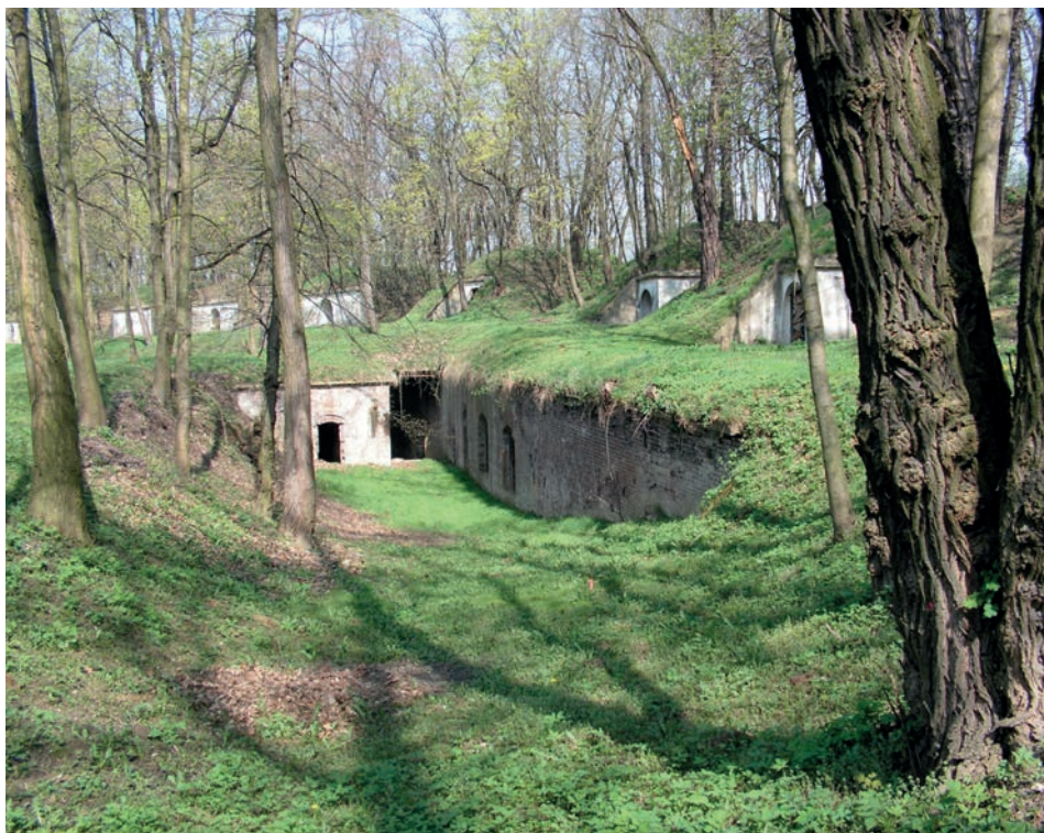
Fig. 3 A vaulted brick shelter located in the inner slope of the embankment – view of the eastern part.
