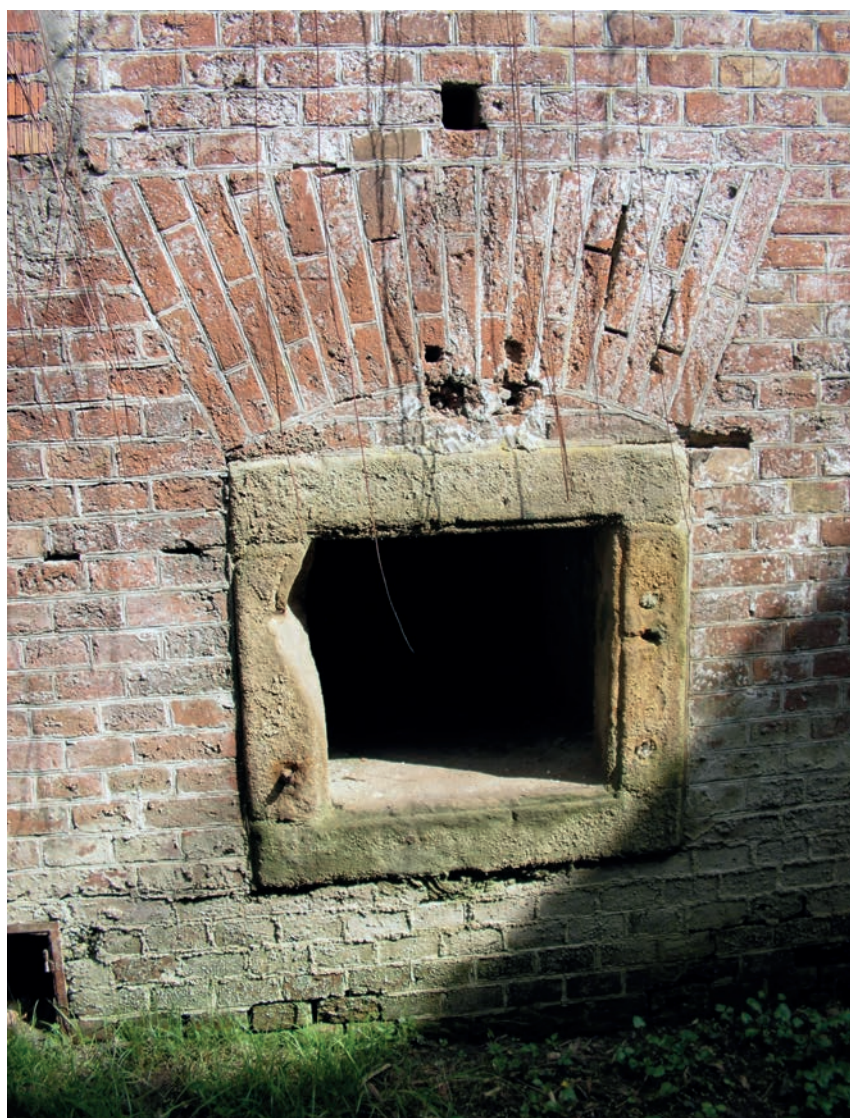
Fig. 18 Sandstone used to finish the window frames.
