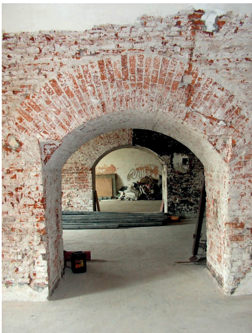
Fig. 12 Enfilade in the interior of the central casemate block.
