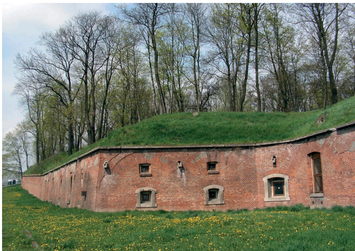
Fig. 7 Neck barracks (neck casserns) – view of the west block.
