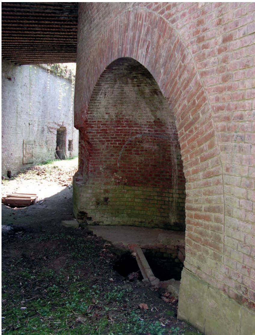
Fig. 13 One of the wells.
