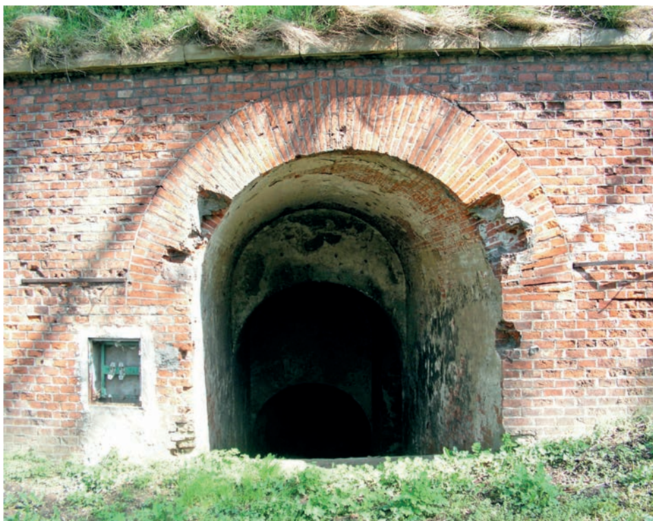
Fig. 4 Entrance to the postern (underground pavements).
