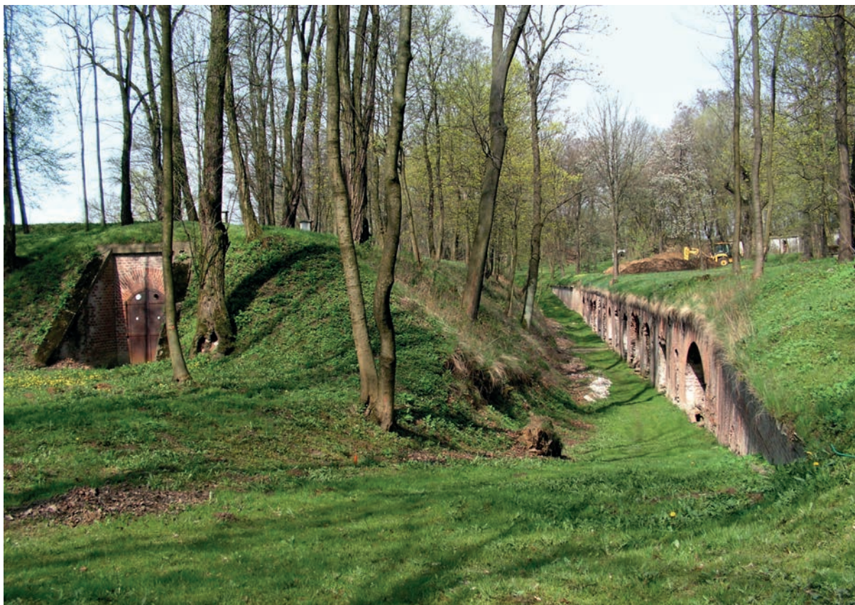
Fig. 9 On the left side a runway gate from the neck barracks, on the right side the central casemate block.
