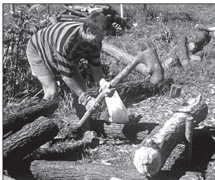
Obr. 14-16 Štipání fošen dřevěnou palicí a kliny. ■ Splitting deals and battens by means of a wooden mallet and wedges. ■
